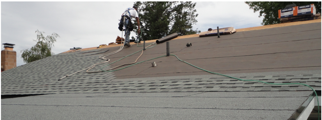
Home construction in Sparks
